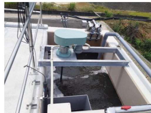
④凝集沈殿槽
